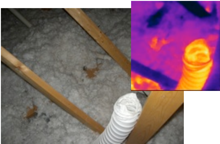
Vent from Hallway bath showing heat loss to attic space from unboxed fan and improper venting throwing moisture into Attic. Could lead to possible mold in Attic
