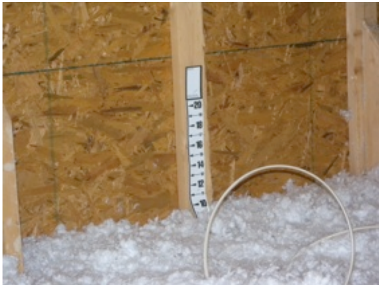
Uneven blown fiberglass in attic. 9" equals approximately R22. DOE recommends between R38 - R60.
