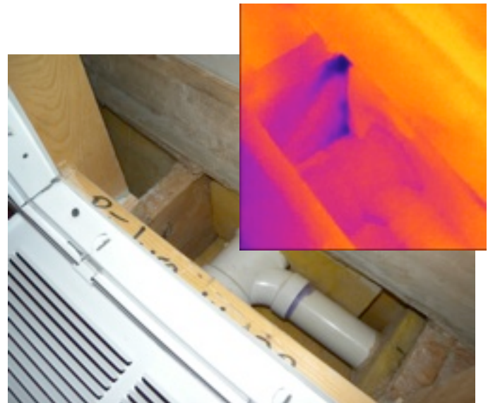
Flow of air in return from unconditioned basement
