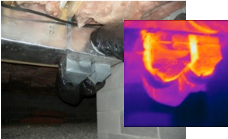
Ductwork in basement showing heat loss
