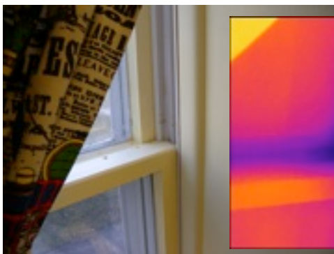
Thermal Bridging at framing members and air movement possibly due to uninsulated rim joists
