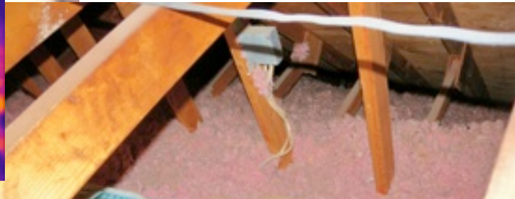
Master Bathroom vent showing heat loss around unboxed fan
