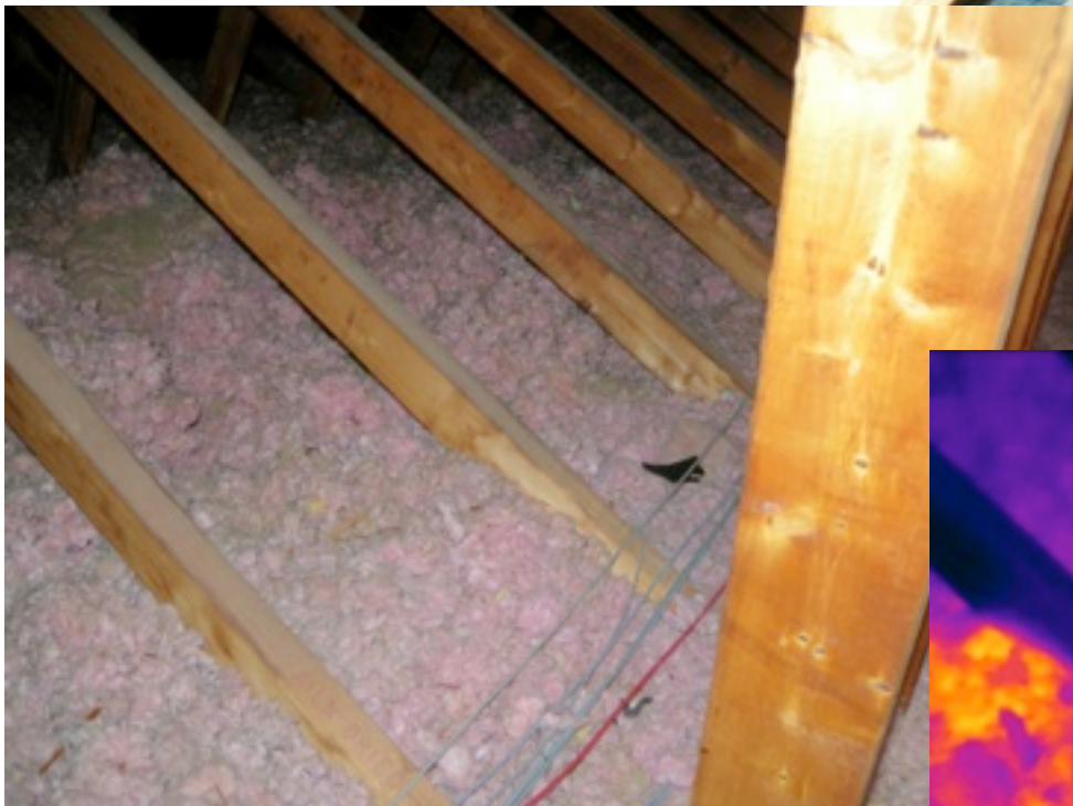
Heat loss into attic around unsealed wire and headers
