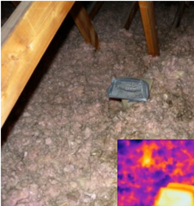
Vent from Hallway bath showing heat loss to attic space from unboxed fan and improper venting
