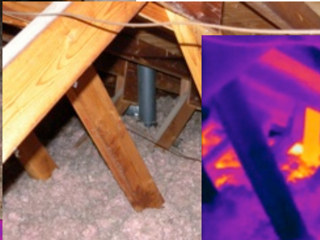
Master Bathroom vent showing heat loss around unboxed fan
