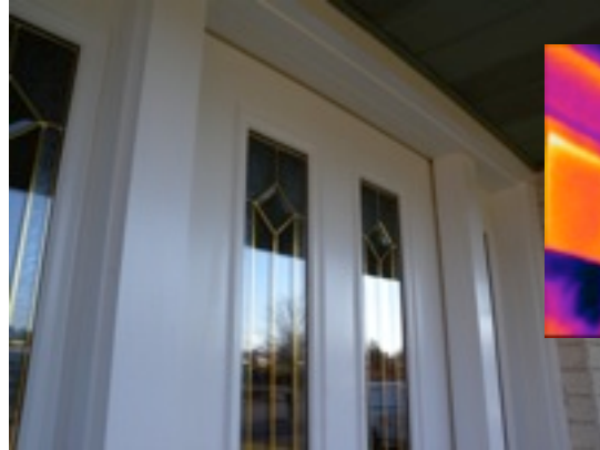
Heat escaping around front door
